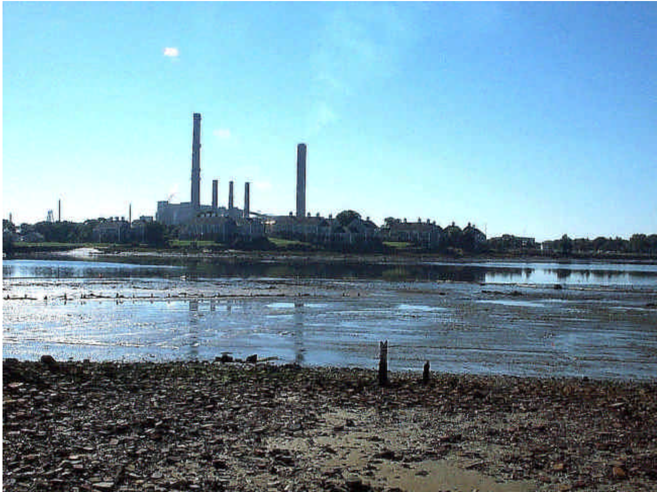
Collins Cove MGP Site
