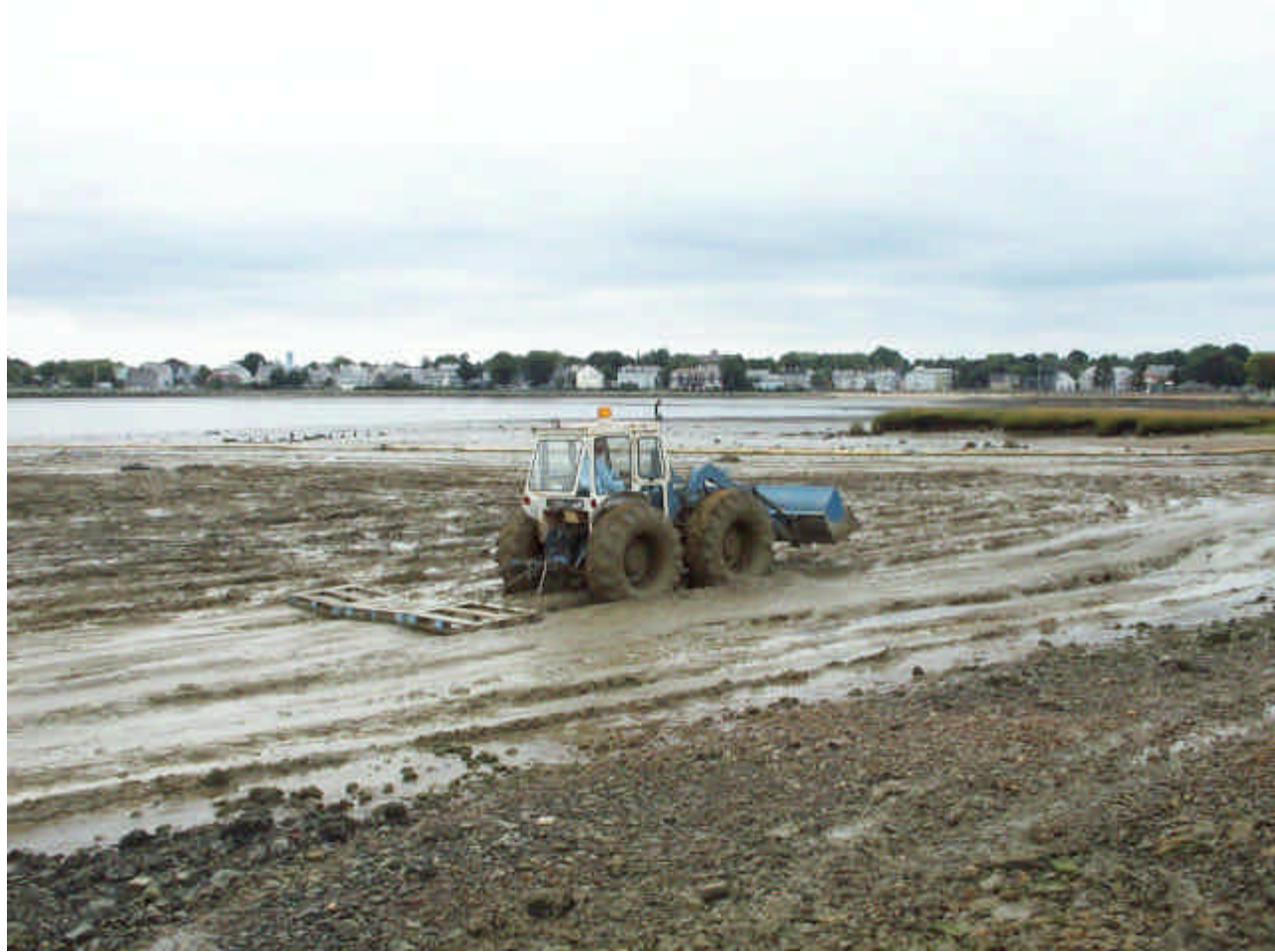
Smoothing of Sediment to Minimize Washout
