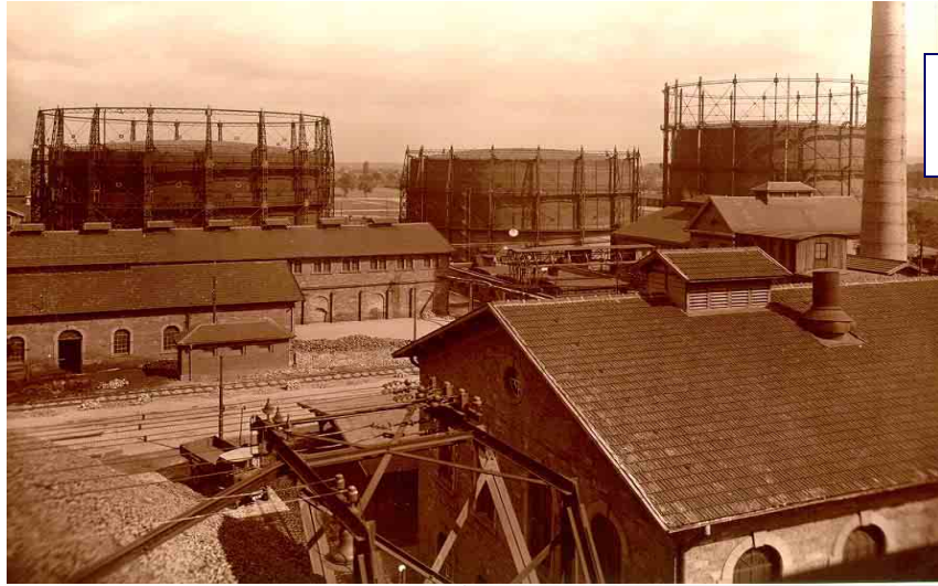
Former gas works plant
