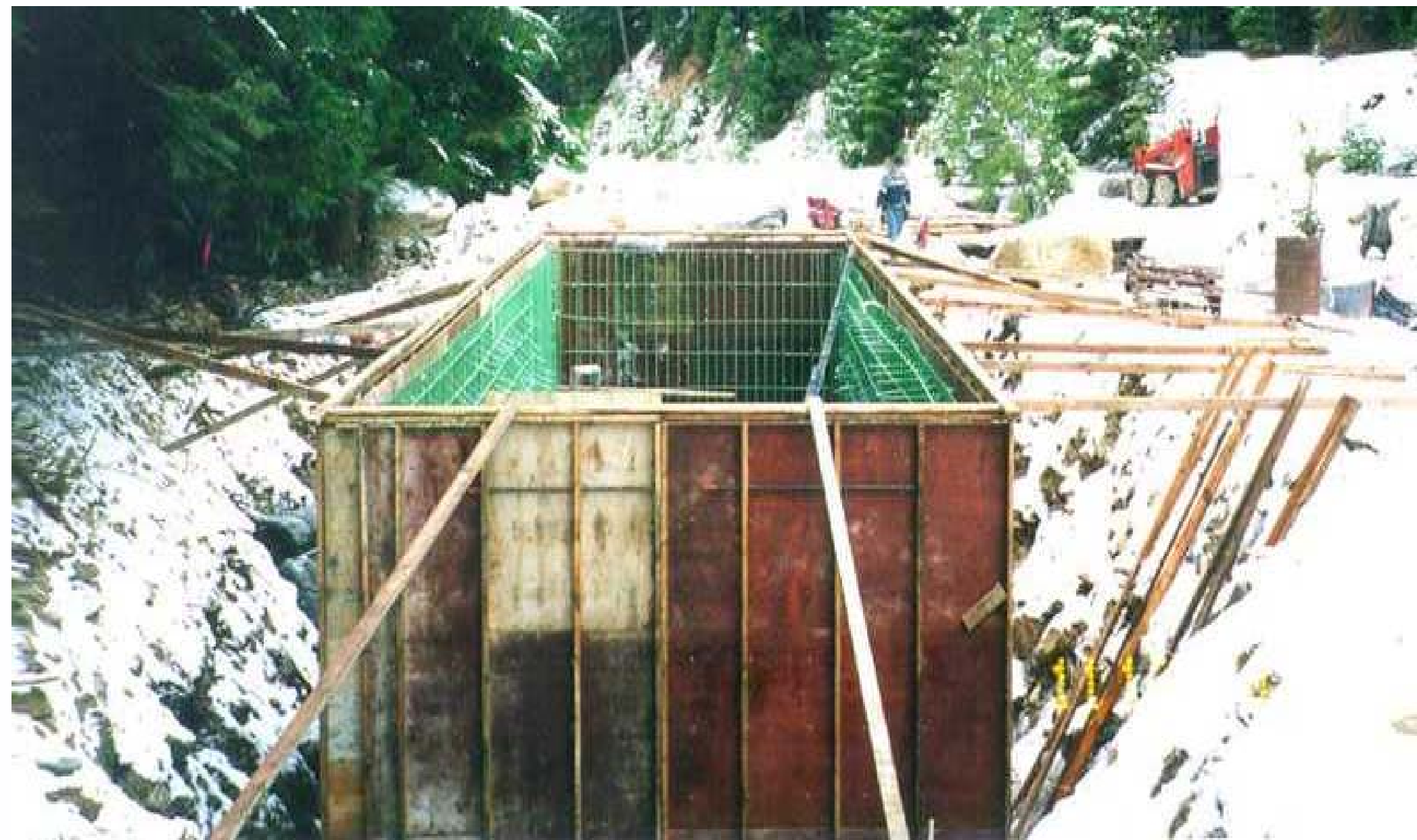
Construction of PRB vault between East Fork of Ninemile Creek and the Tailings Pile.
