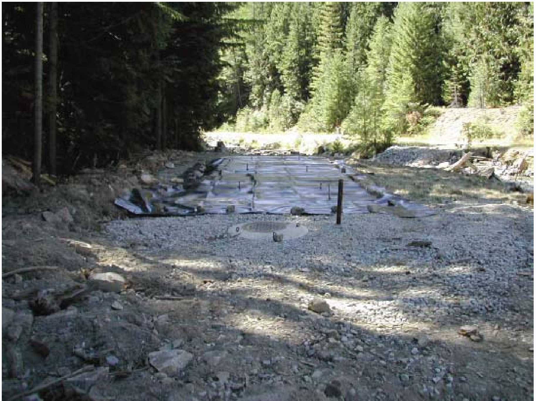
Completed PRB vault at Success Mine. Flow is from bottom of photo to top and into Ninemile Creek behind.
