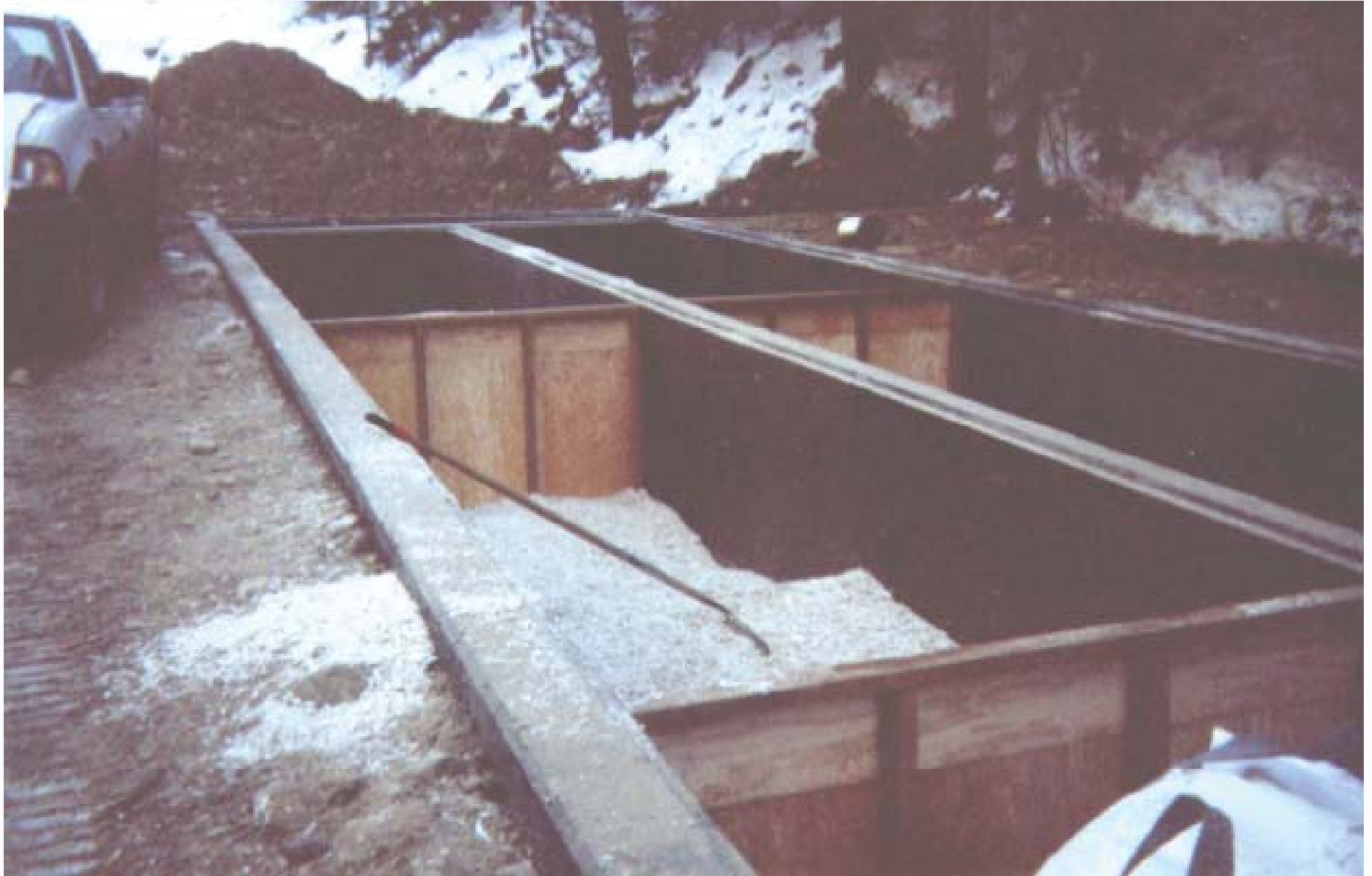
Installation of the Apatite II in the baffles of the PRB vault.
