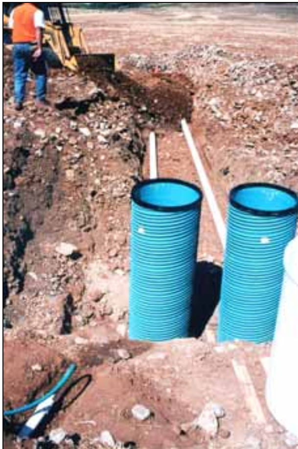
Dosing siphon measure drainage
