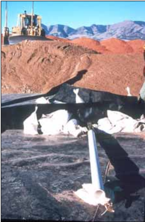
HDPE drainage collection system
