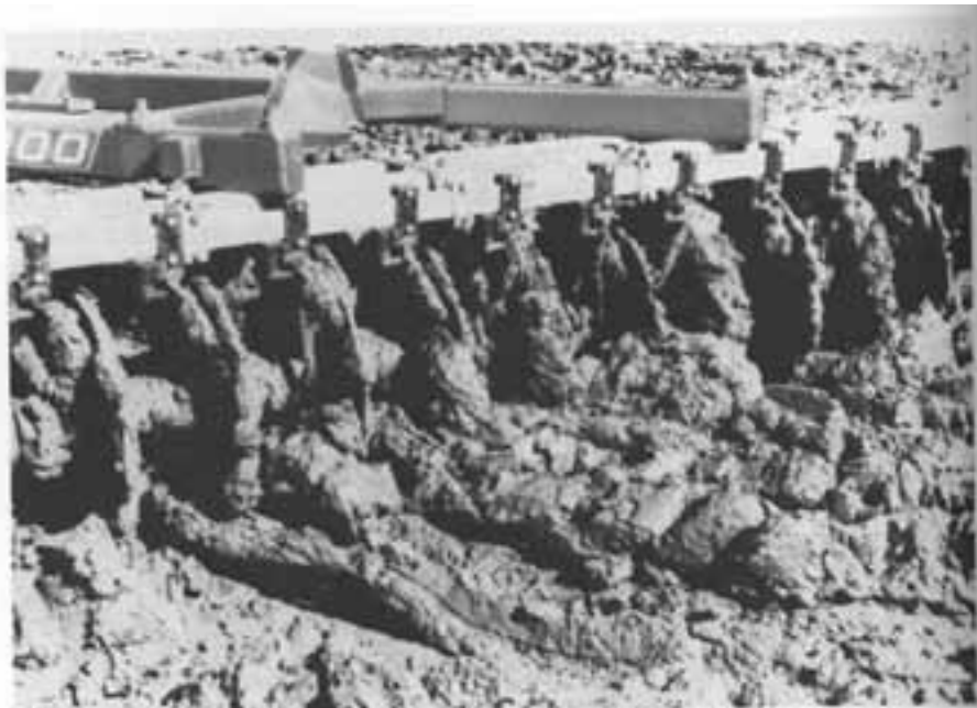
Figure 15-11 Used for high solids stabilization not requiring high-energy mixing. (Harmon Environmental Services, Inc.)
