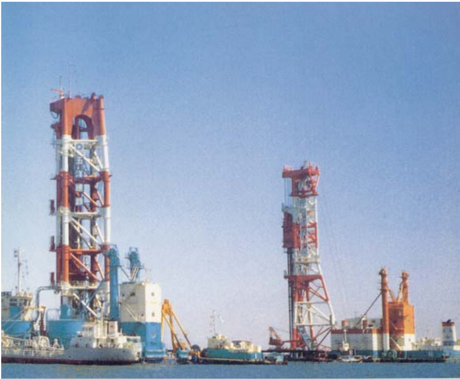
Sea Floor Stabilization in Deep Water
