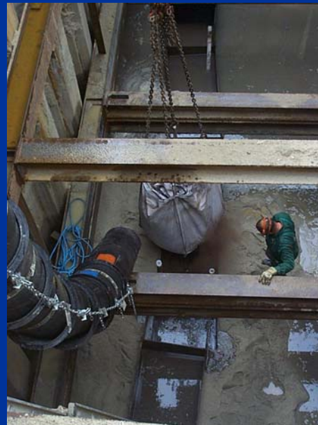
4) Filling of 270 ton of the Fe 0
