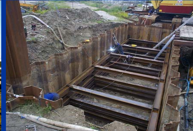
3) Construction of a metal frame for filling of the Fe 0
