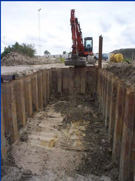
2) Removal of the soil & water from the case
