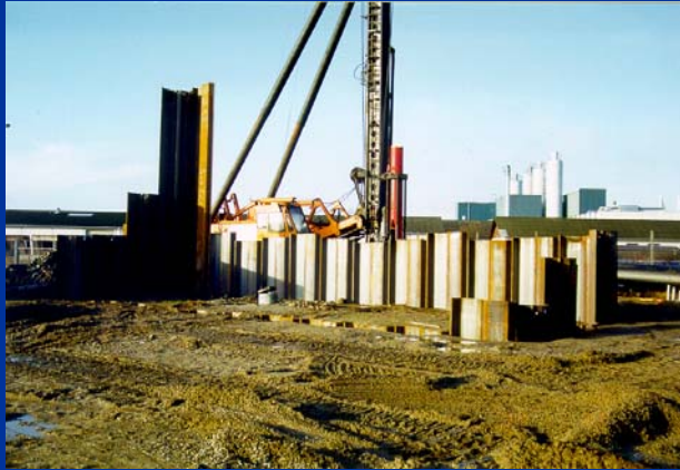
1) Ramming down of the sheet piling case
