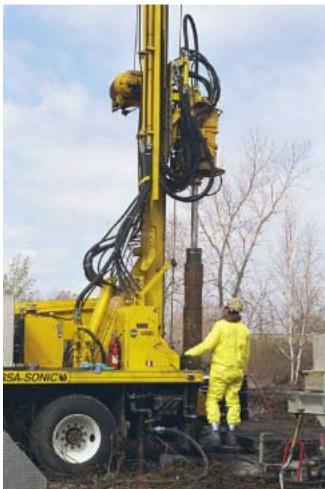
Rotasonic drilling
